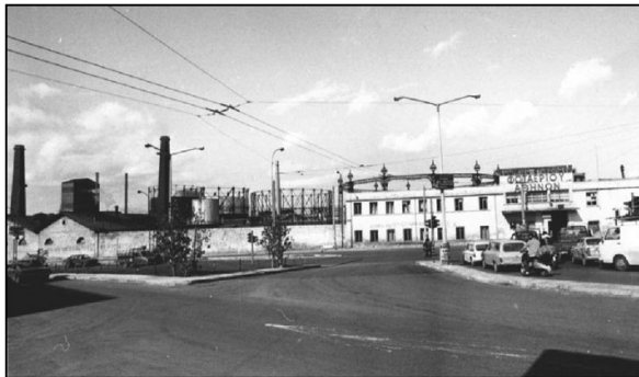
Figure 3: The ‘Gas Works’ facilities.
